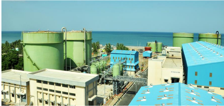
FIGURE 18: Nemmali seawater desalination plant located at the coast of Bay of Bengal in Chennai Nagar (Kalaivanar Nagar Pond) and J J Nagar Lake. 102 A study should be conducted to check these waterbodies' revival potential and use them as drinking water sources.
